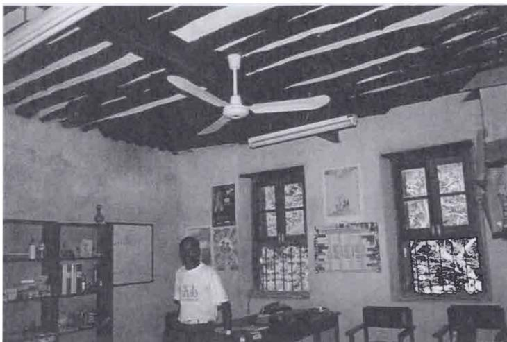
*Fig. 6: A steel beam instead of a wall supports the ceiling load.
